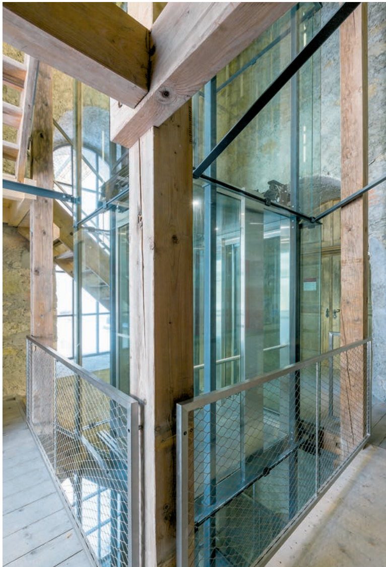
The architect sought to achieve maximum transparency when integrating the lift into the wooden stairwell.
