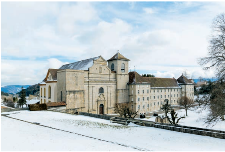
A new lift is concealed in the north tower of Bellelay Abbey Church.
