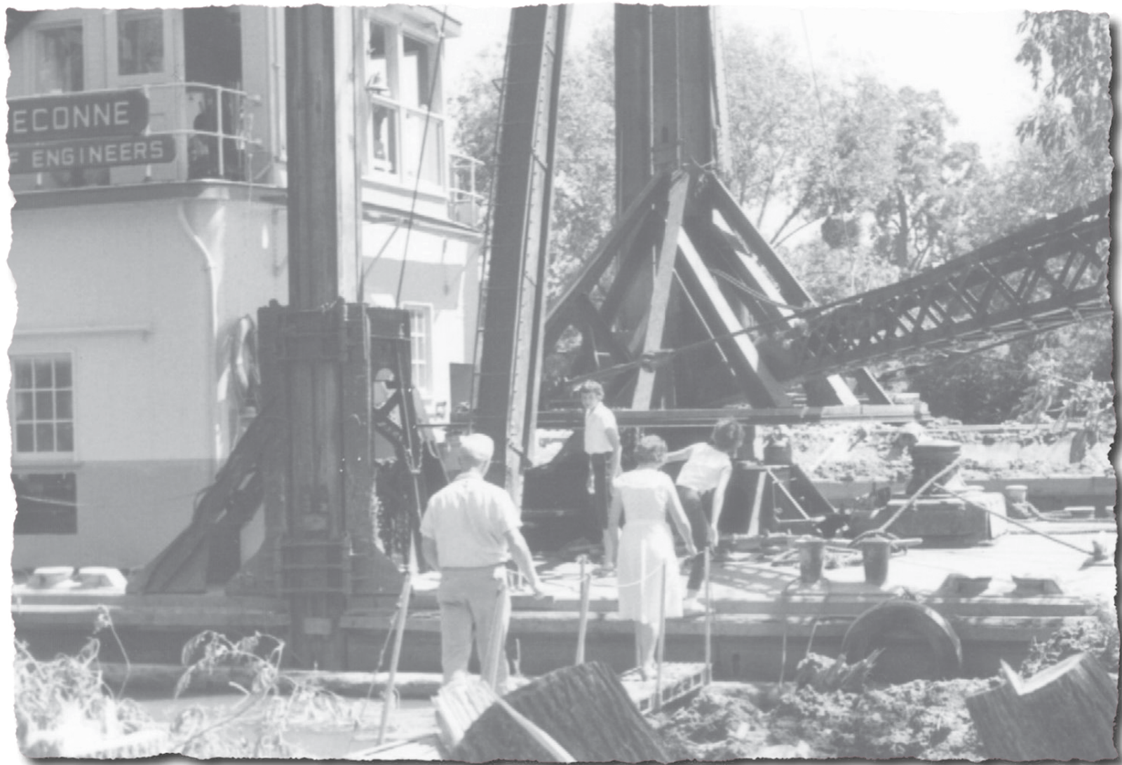
Dredging of Brothertown Harbor • August 1962
