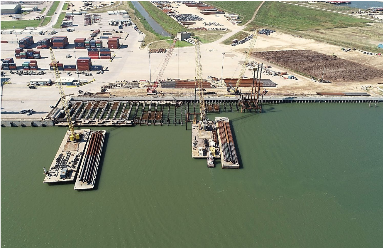
Photo Caption: Completion of Reach 3 of the Freeport Harbor Channel Improvement Project
